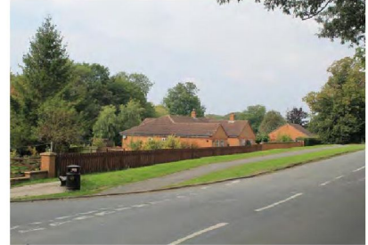
View northwest towards the sites boundary from Langton Road
