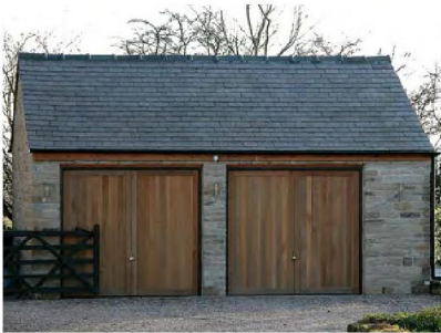
Typical Image: Courtyard and adjoining garage
